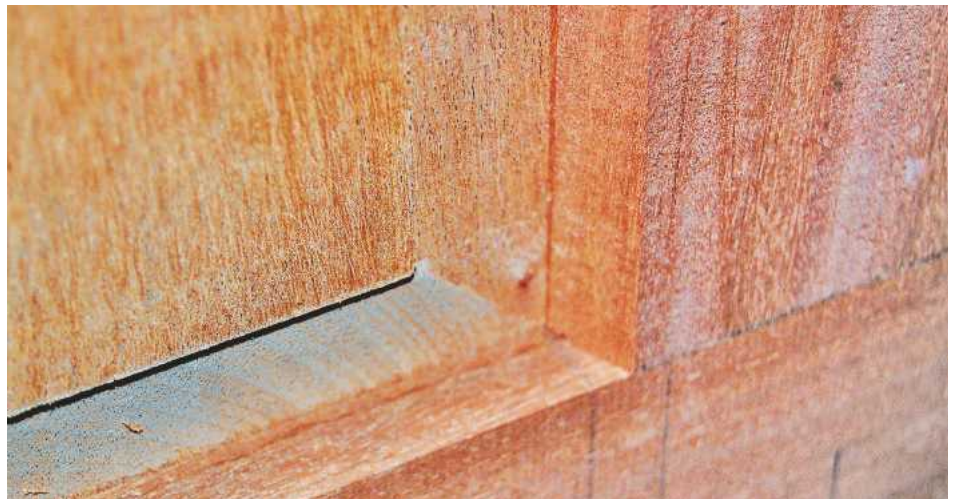
▲ Pic.22 Note the chamfer on the bottom rail and raised panel
